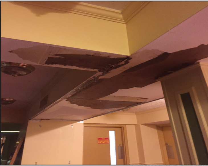
SUBMITTED BY SYDNEY BEAVERS Ceilings destroyed in Clark Hall from water line bursting on the third floor.
